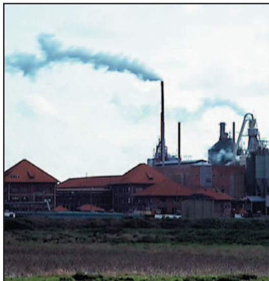
The "smoke" from this factory's chimneys consists primarily of water vapor and carbon dioxide, two products of the combustion of fossil fuels.
